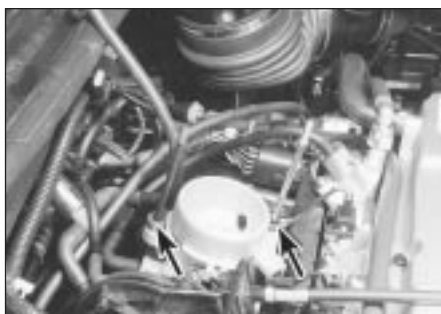
4.10A Lift plenum chamber and (where fitted) disconnect the vacuum hose - note the two rubber spacers (arrowed) . . .
